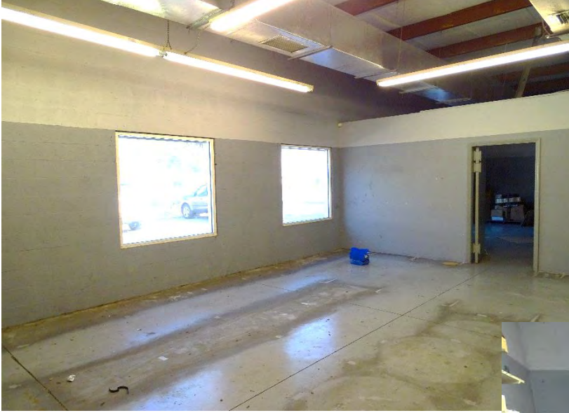
Ample Storage Areas at Sides and Rear of Shop Floor
